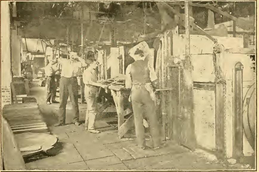
HARDENING AND TEMPERING HAND SAW BLADES
