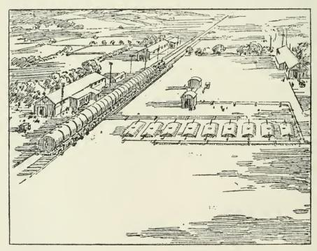
Railway Tank Train pumping into Pipe-line.
