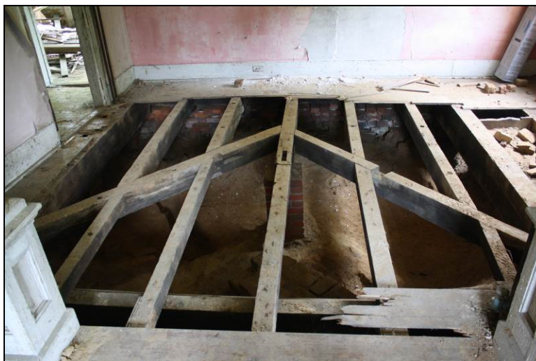
Figure 8-6. Dragon beams with later infill sub-joists.
