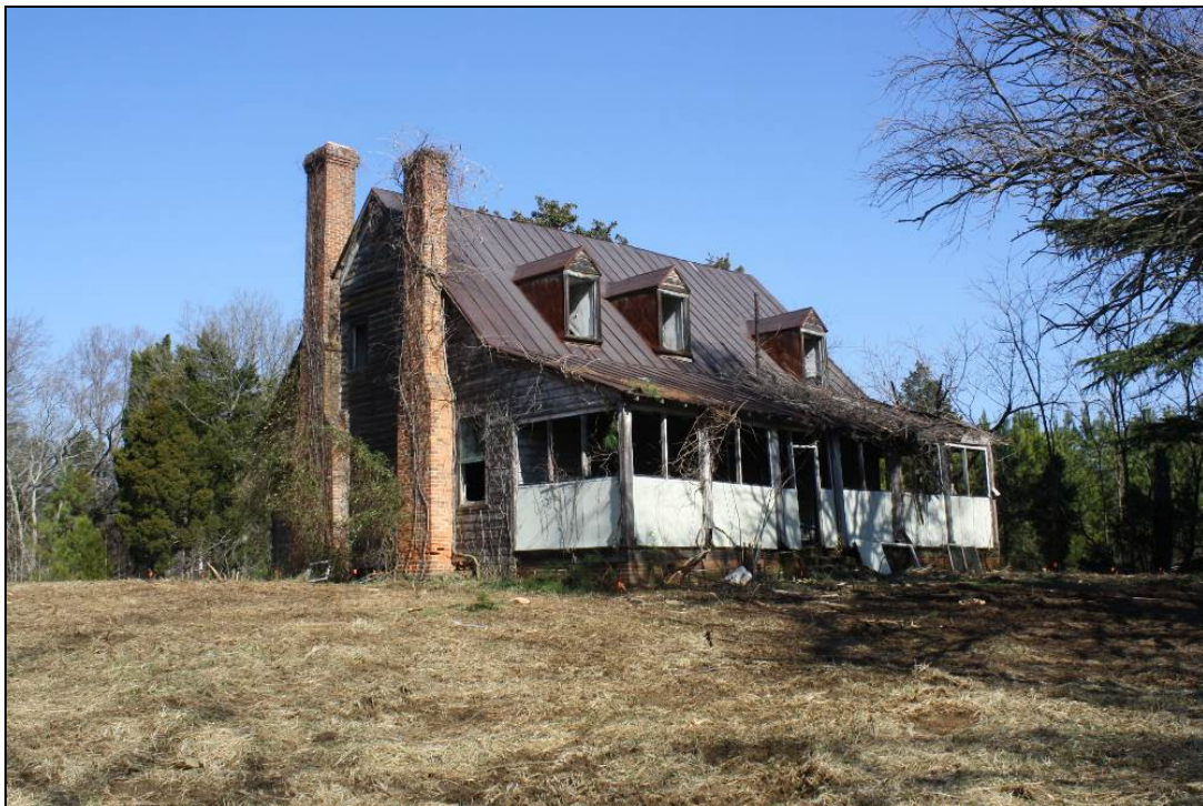
Figure 8-1. Spring Hill house, front and west side
