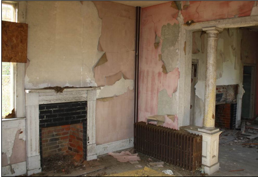
Figure 8-32. Matching fireplaces in first floor rooms.
