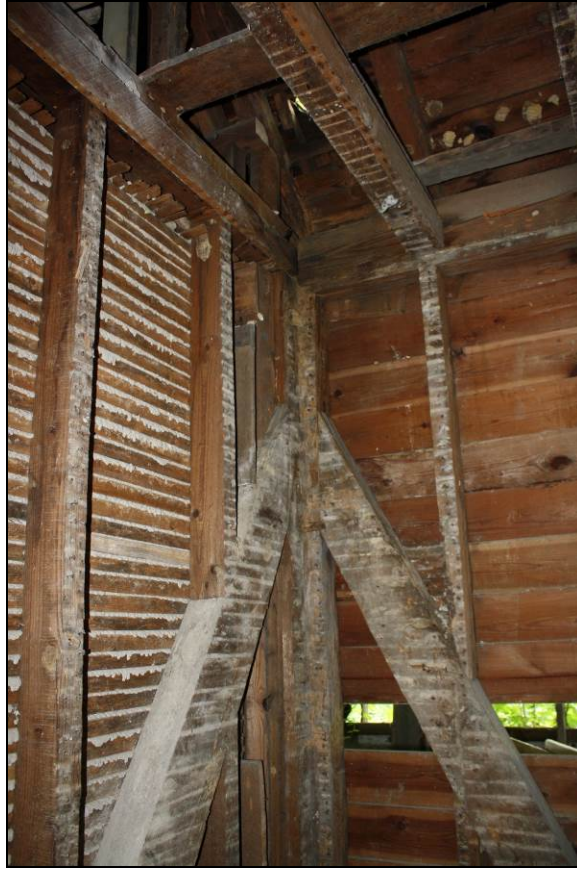
Figure 8-7. Guttered corner post and down braces.
