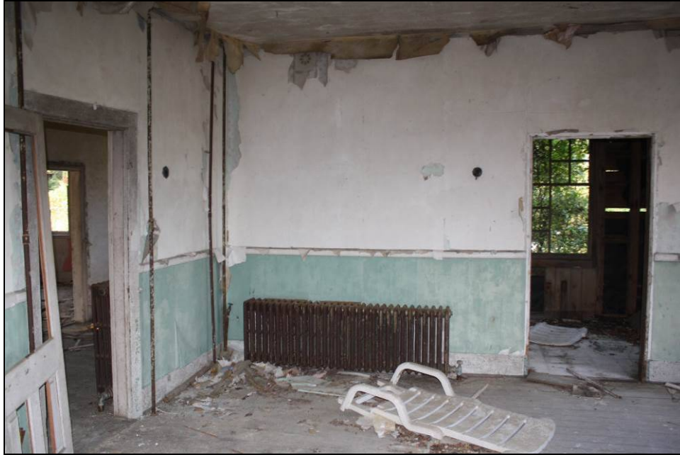
Figure 8-19. Dining room in addition with enclosed porch to rear.
