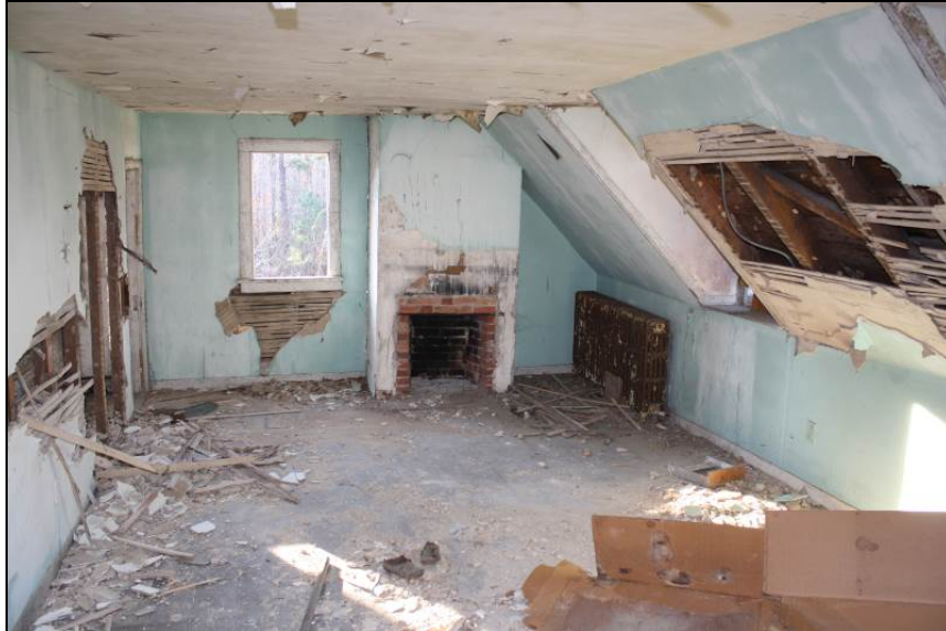
Figure 8-21. Northern bedroom with fireplace.
