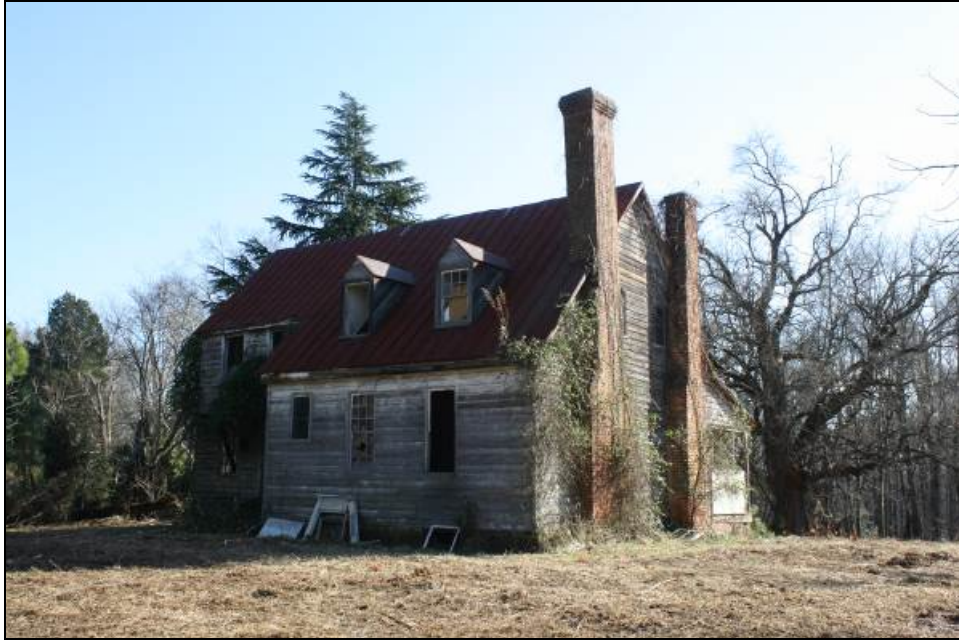
Figure 8-15. Fenestration on original block.
