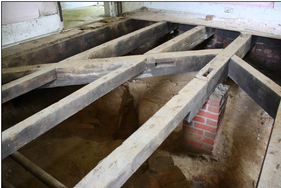
Figure 8-5. Brick piers reinforcing framing over removed internal chimney
