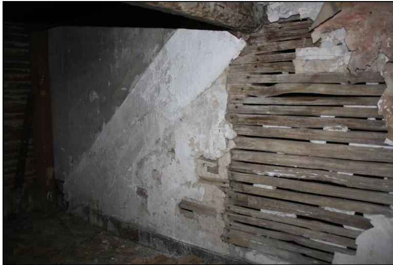
Figure 8-26. Original split pine lath under stair landing.
