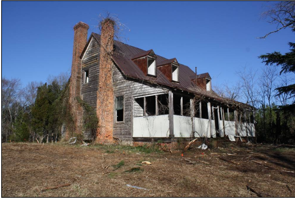
Figure 8-13. Full-width front porch.
