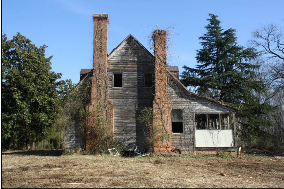
Figure 8-11. West side end chimneys.
