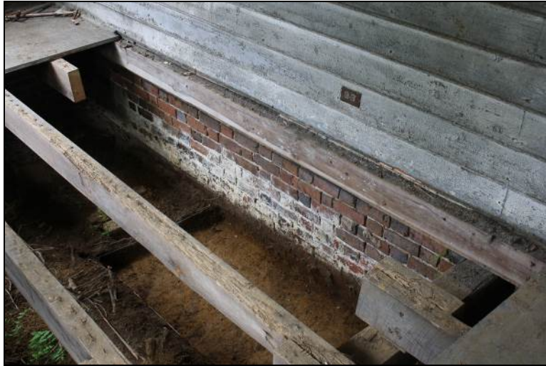
Figure 8-2. Original foundation laid in Flemish Bond
