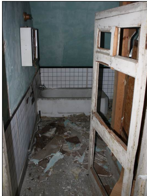
Figure 8-22. Bathroom in southeast room.
