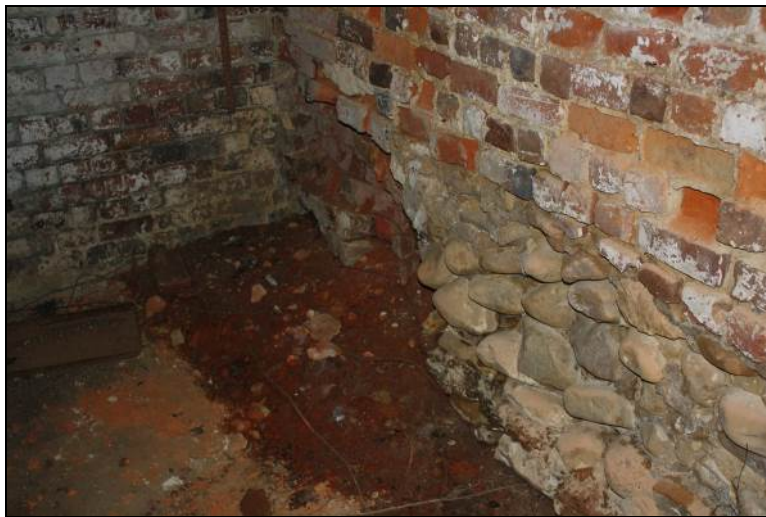
Figure 8-3. Cobbles in cellar wall
