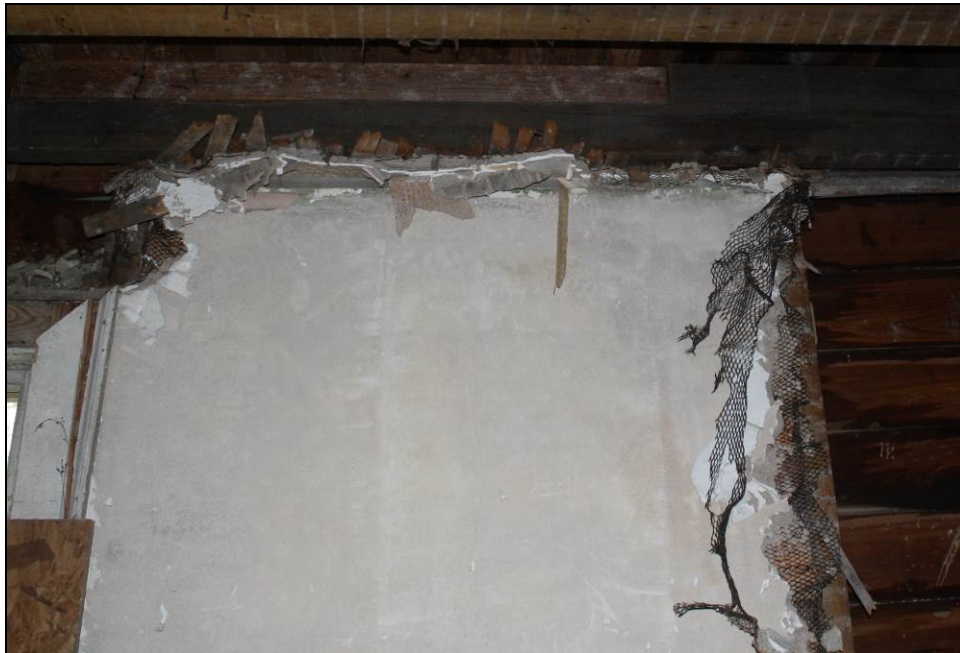
Figure 8-27. Remnants of metal lath under plaster on 1925 chimney.
