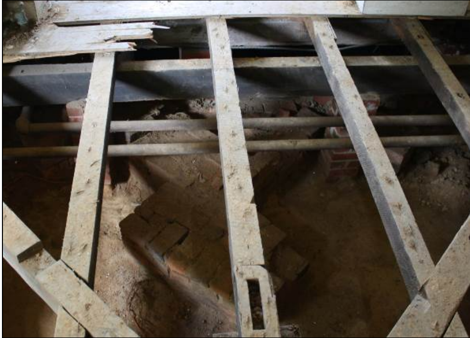
Figure 8-4. Original interior chimney base
