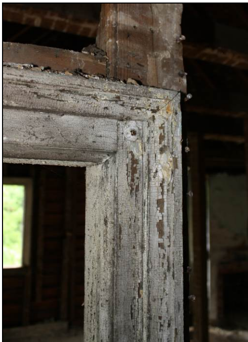
Figure 8-29. Greek Revival molding on original door frame.
