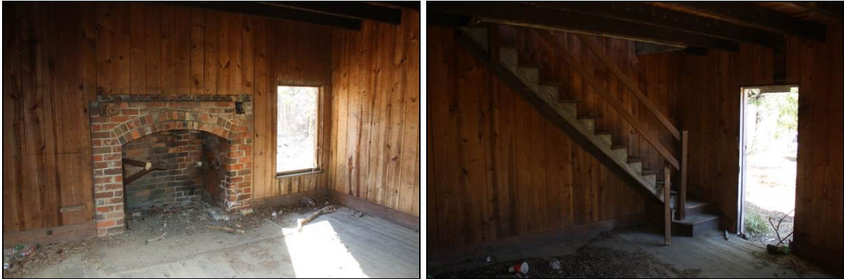
Figure 8-34. First floor fireplace (Left) and stairs (Right) in the kitchen outbuilding.
