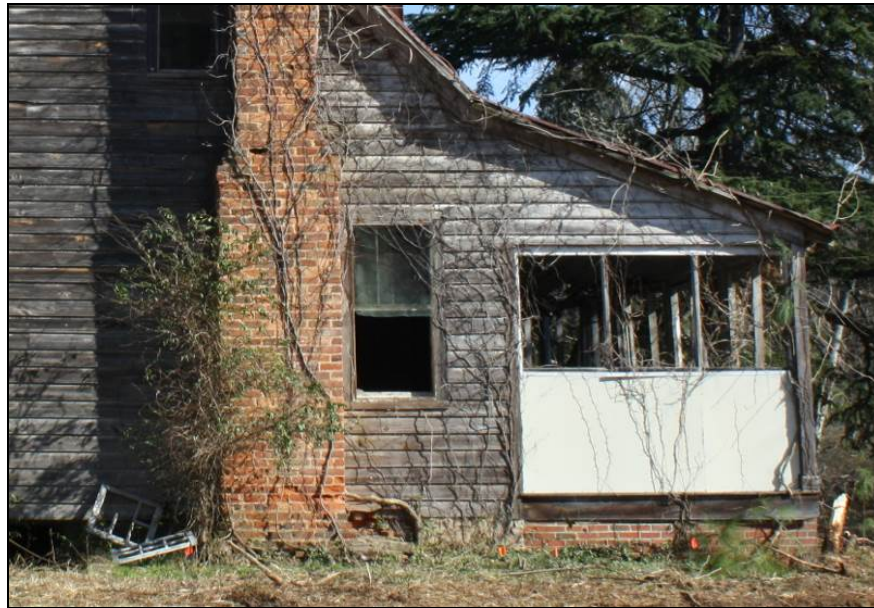
Figure 8-31. Window added to west side.
