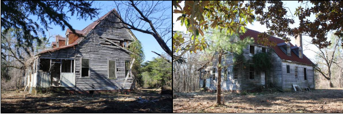
Figure 8-10. Gable roof over wing Addition, 1.5-story on front (Left) and 2-story on rear (Right).
