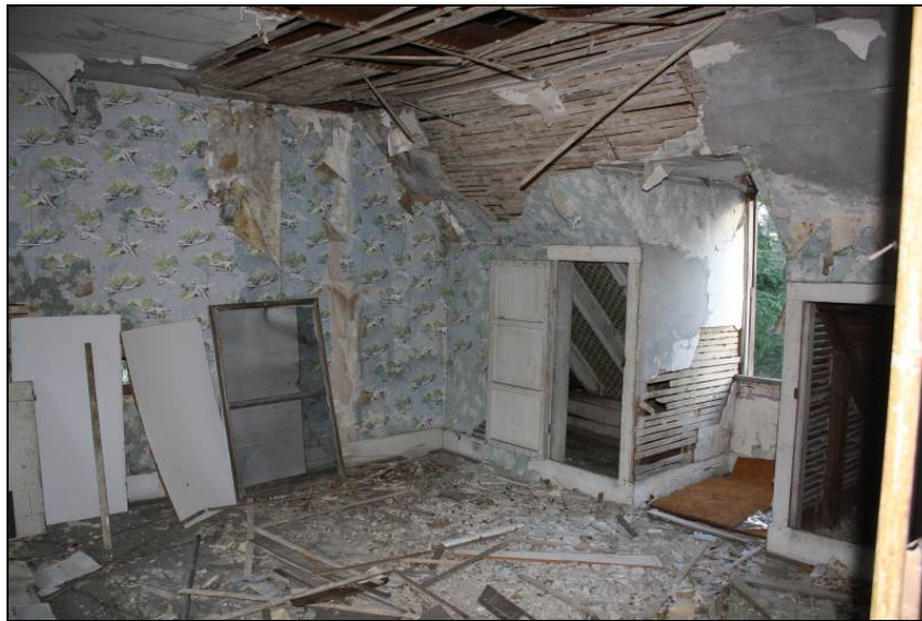
Figure 8-24. Bedroom in wing addition.
