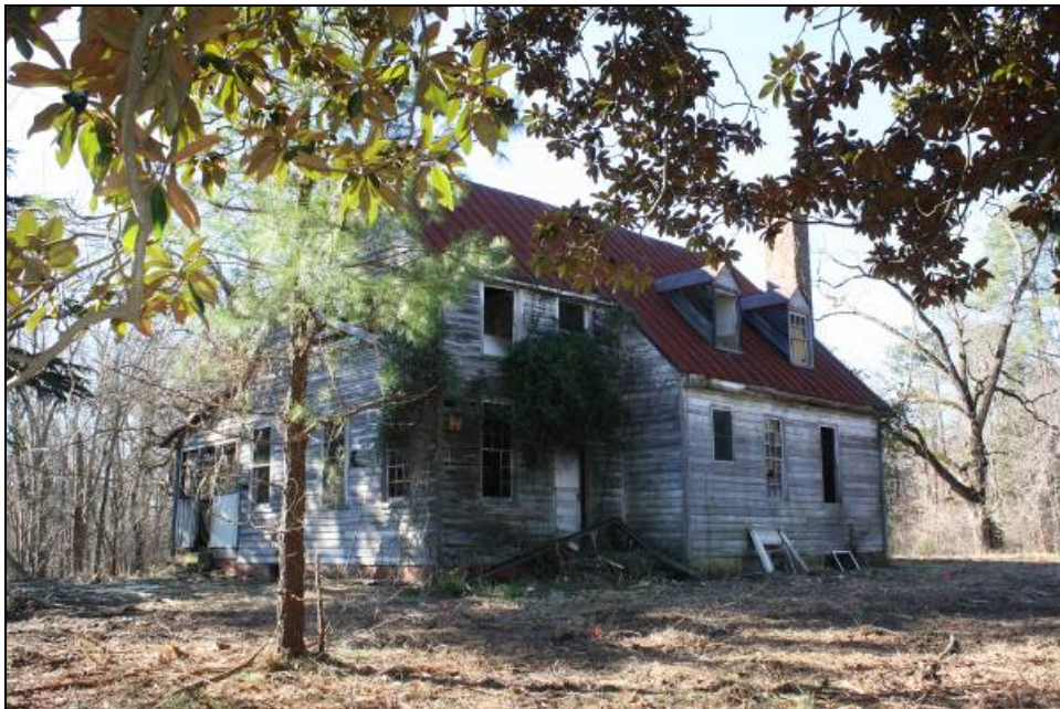
Figure 8-16. Fenestration on wing addition.
