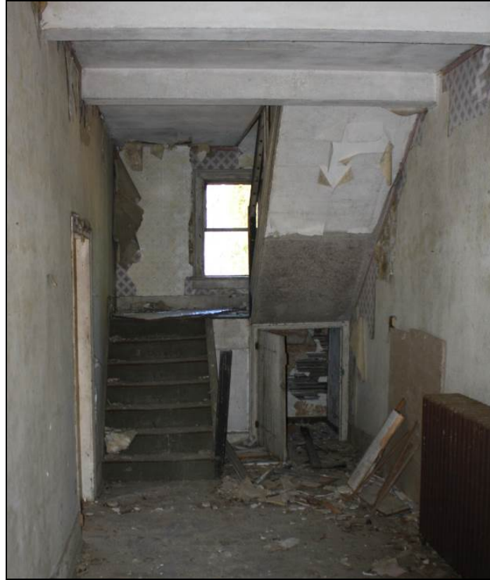
Figure 8-20. Stairway at end of side passage.
