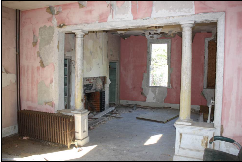
Figure 8-17. Partition wall with columns on knee walls.
