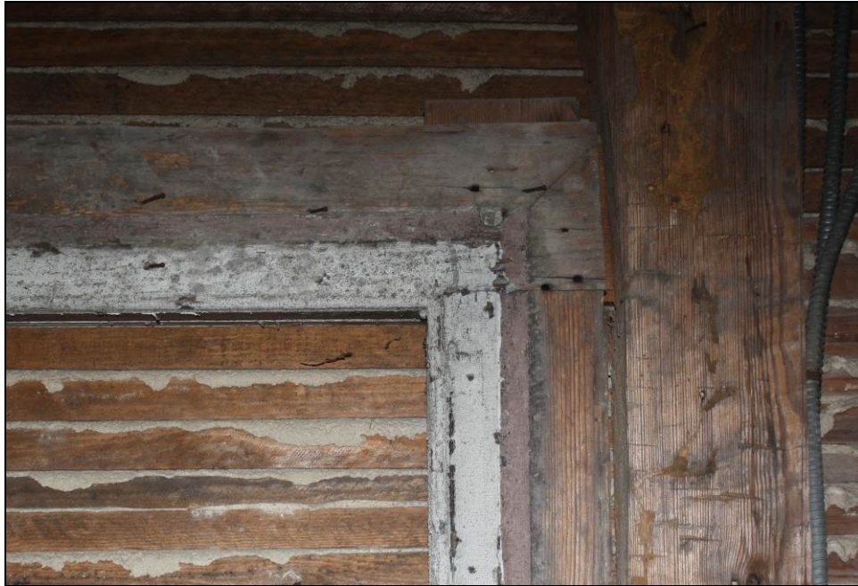
Figure 8-28. Detail of original pegged door frame.
