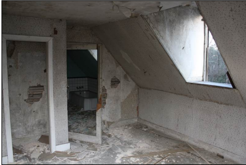
Figure 8-23. Bedroom in southwest room with door to bathroom.
