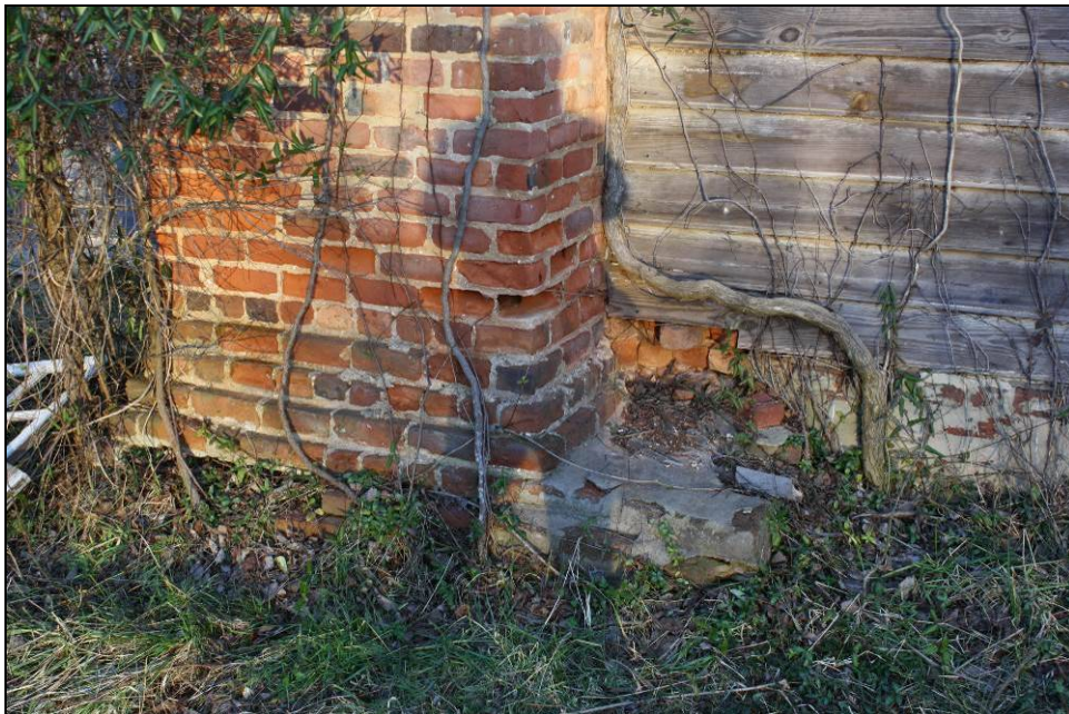
Figure 8-12. Southern end chimney with replacement stack over older base.
