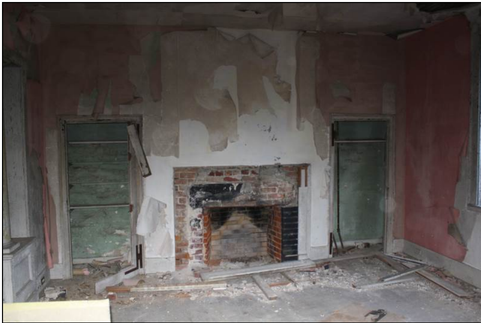
Figure 8-18. Fireplace in northern room with flanking closets.
